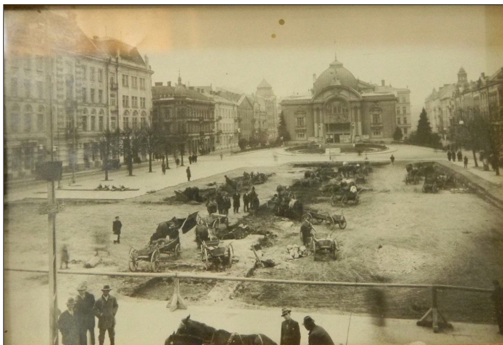
Works on central part of Vasile Alexandri Square deepening. (From Chernivtsi Regional Museum of Local Lore)
